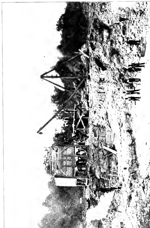
Arrangement of Crushing Equipment—Stone in quarry buckets is raised by a crane to a platform above hopper leading to Crusher.
